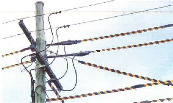
Figure 16 – Tiger tails fitted to overhead power lines
