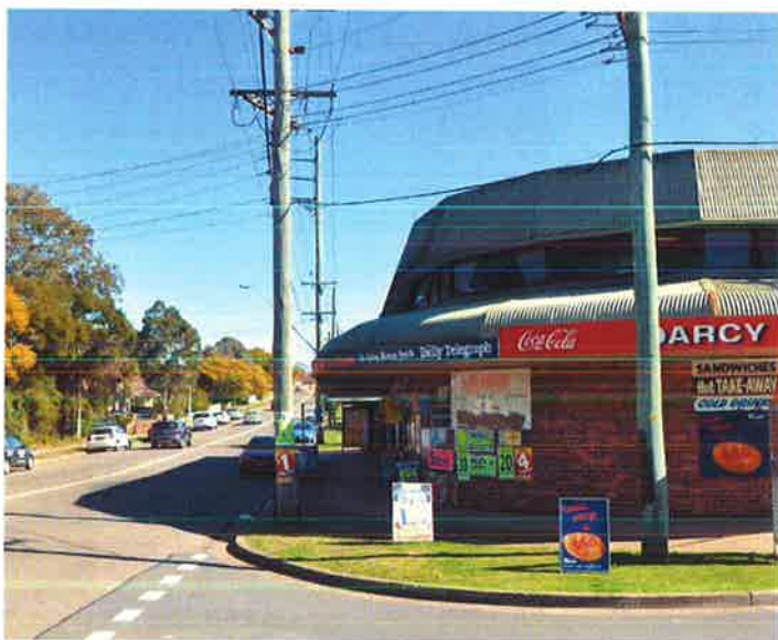
High and low voltage overhead mains
